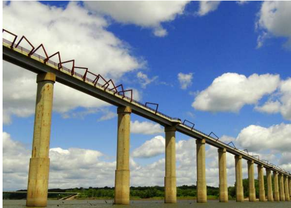
High Trestle Trail Bridge
